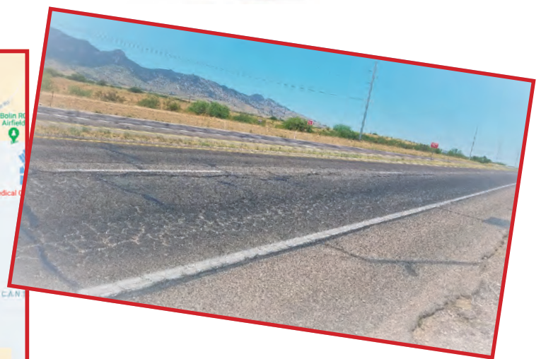
Buffalo Solider Trail disintegrating roadway surface
